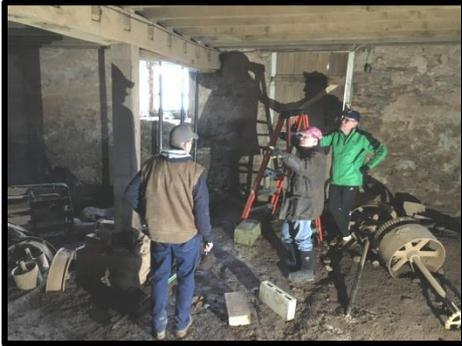
**Swigart's Mill** has a widespread infestation of powder post beetles in the flooring and beams and will need to be thoroughly treated. The back porch has serious deterioration (again) and must be repaired, many areas of the interior stucco/plaster are failing (and falling), and the stone foundation has major issues. Richard Fox, Mike Loges, and I recently installed multiple floor jacks in the basement
